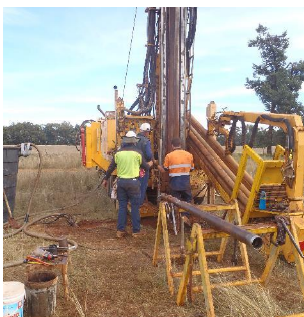
Diamond core drilling
